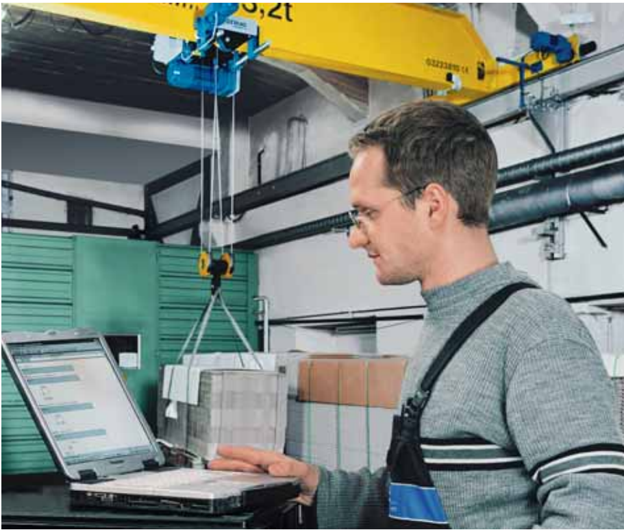
Crane system data can be displayed for preventative and scheduled maintenance
