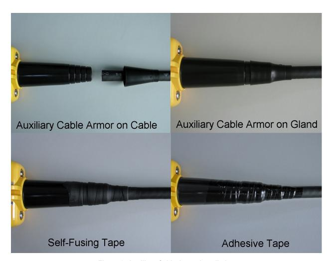
Figure 2: Auxiliary Cable Armor Installation
