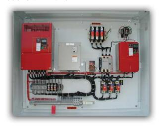
Magnetek's custom control panels with IMPULSE•G+ and VG+ Series 3 Drives provide the ultimate solution for overhead material handling. Built and designed to your specifications, these panels include all the standard features of our pre-engineered panels, and can be custom designed to your exact specifications. Our experienced engineering staff provides technical support and extensive overhead material handling expertise when quoting your project.
