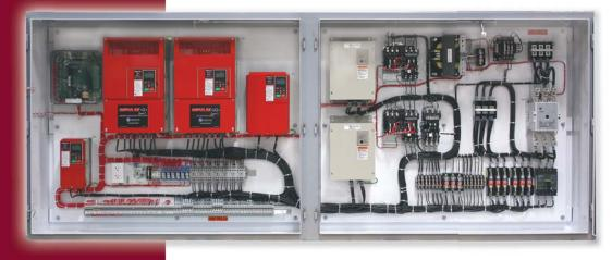
Magnetek offers pre-engineered or custom engineered panels featuring our high quality components designed for your specific application requirements. For specialized and unique applications, custom panels are designed and built to your specifications.
